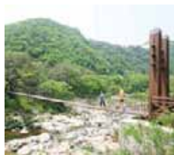
Dutayeon suspension bridge
