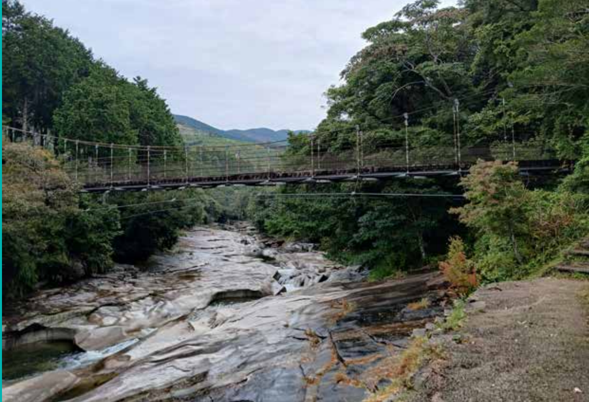
The 70-meter suspension bridge.
