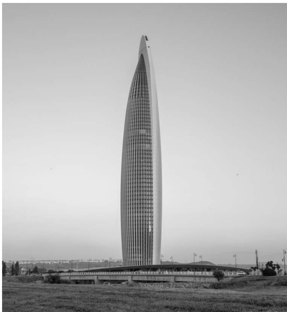
Mohammed VI Tower is the tallest building in Morocco and one of the tallest in Africa.
