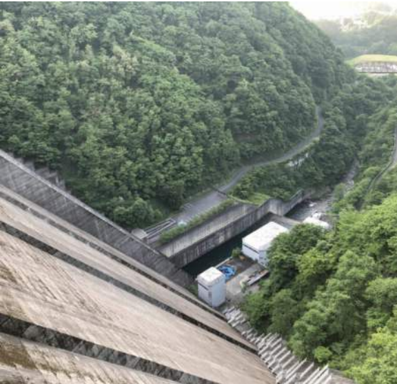
The vew from atop Urayama Dam in Chichibu, Saitama prefecture, Japan, can be a dizzying sight.
