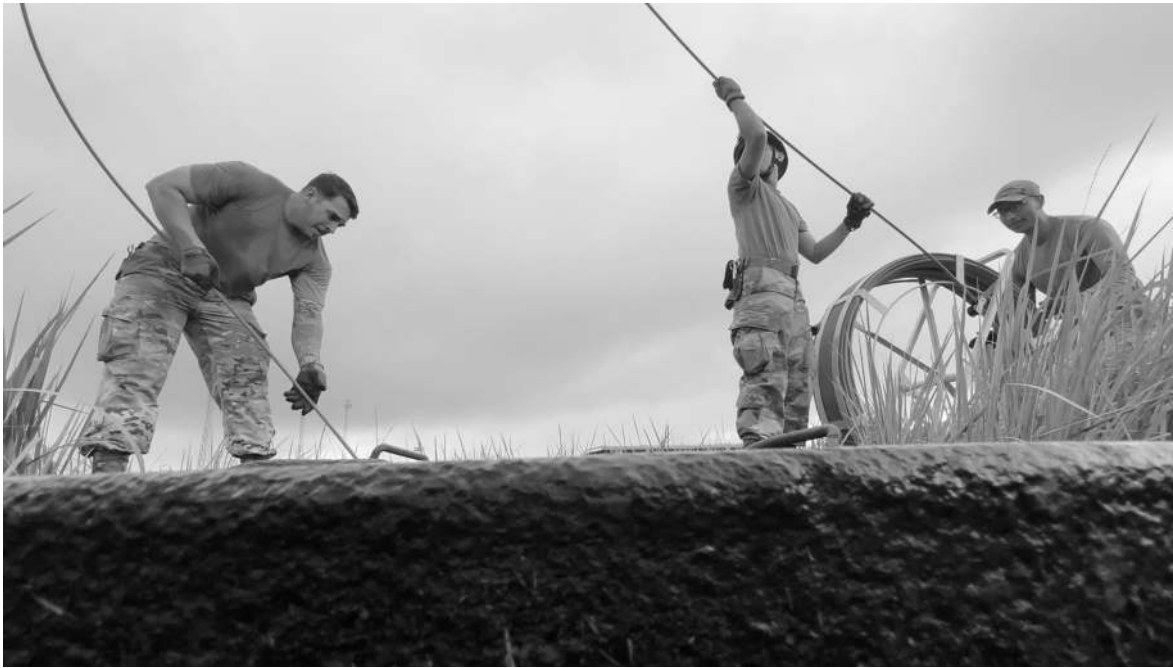
Air Force Staff Sgt. William Johnson, left, Airman 1st Class Gabrielle Oropesa and Senior Airman Carlos Reye feed a pull string into a duct rodder while replacing underground cable at Yokota Air Base, Japan, last month.
