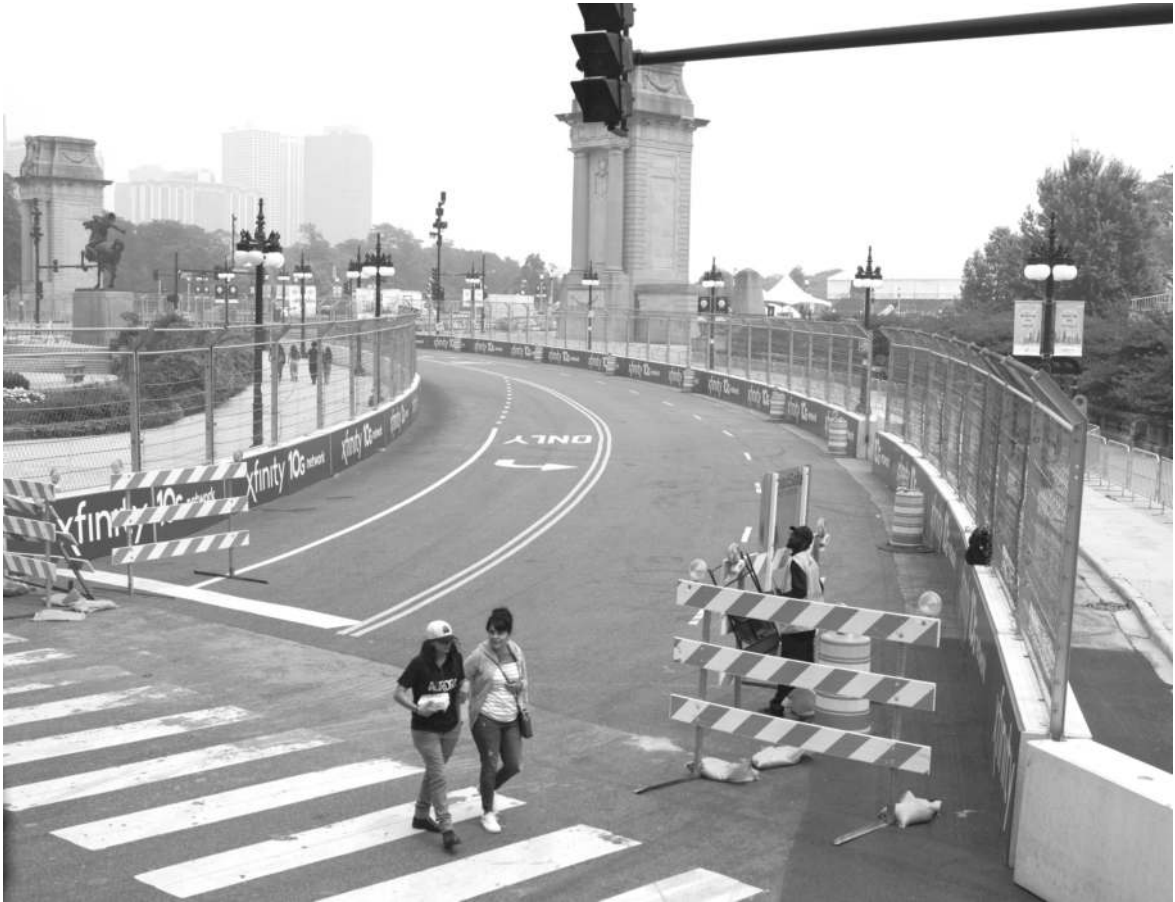
Construction goes on at East Congress Plaza Drive on Tuesday for the NASCAR Cup Series race in Chicago.
