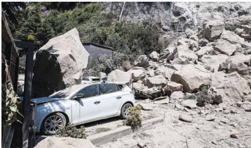
A view of the damage caused by the earthquake that struck Pozzuoli.
