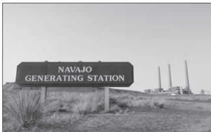
The coal-fired Navajo Generating Station, which will close by the end of the year, is shown on Aug. 19.
