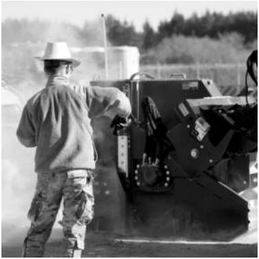
Krawczyk acts as a ground guide while wheel saws are used to remove a patch of damaged concrete.
