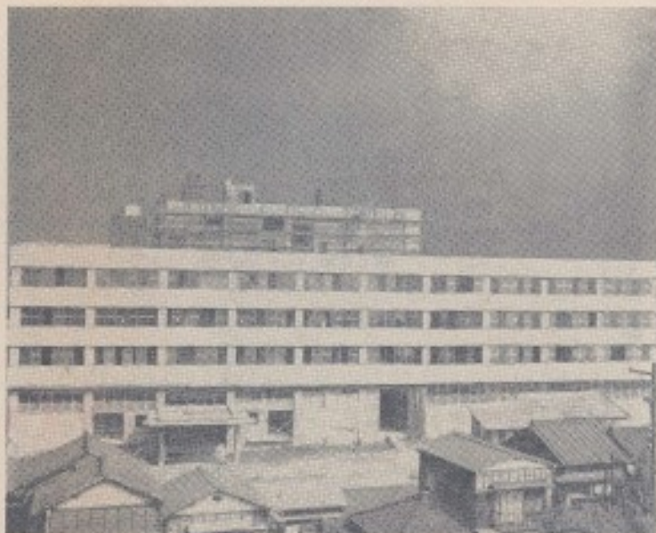
New home for the paper is this nearly completed four-story building near old home.
