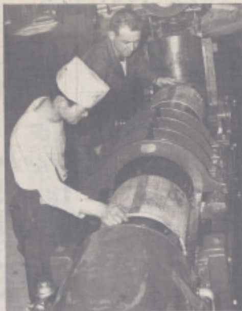
. . . and the type was placed in a 'form' (left). Under five tons of pressure the type was impressed onto a mat, which was used to create a plate (above) for the printing press. Today, high-tech equipment has streamlined the printing process.
