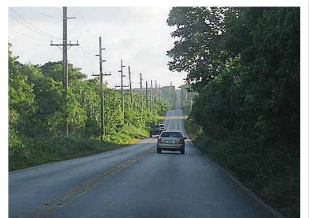
Route 15, commonly referred to as the "Backroad" provided an undisturbed link from Mangilao to the back gate of Andersen Air Force Base in Yigo. Several houses have sprung up along this once sparsely populated road. Photo by Nathalie Pereda, Courtesy of Guampedia
