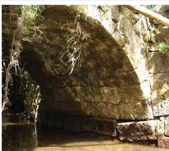
Taleyfac Spanish Bridge
