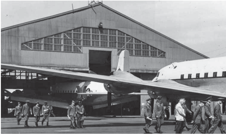
This undated Air Force photo shows Building 800 at Yokota Air Base. Photos by U.S. Air Force
