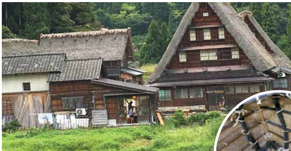
Built without nails, the flexible joints of pillars and beams are resilient enough to withstand the large amounts of snow falling.
