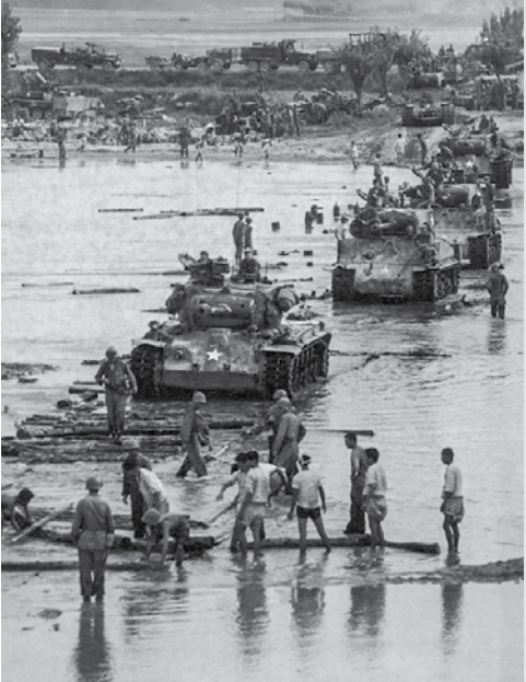
A U.S. Army M26 Heavy/Medium Pershing tank leads, followed by a pair of M4A3E8 Sherman tanks and another M26 Pershing and support vehicles, as the column moves across the Hwanggang River on logs placed on the riverbed with the aid of Korean laborers. Photo by Edwin T. Tarr, DOD
