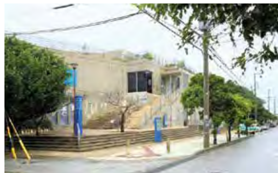
Tsushima Maru Memorial Museum is designed like the ship itself, you board on the upper deck and descend below the decks.
