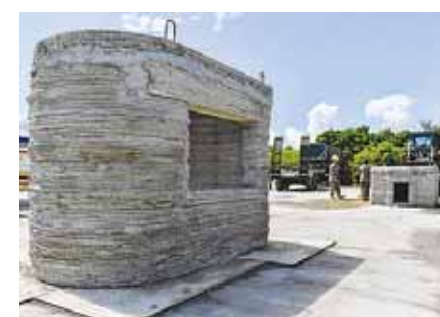
Concrete printing technology created these structures at Camp Hansen.
